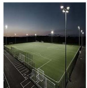
Typical 3G Artificial Grass Pitch (AGP) Installation
